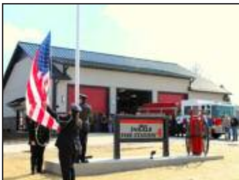
A new fire station for DeKalb County.
